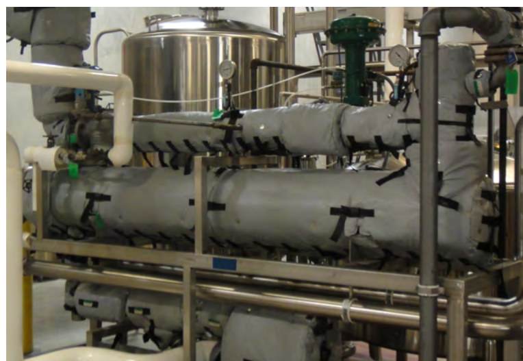
STEAM PASTEURIZING HEAT EXCHANGER PIPING & FITTINGS Design: LT500LFP – Food grade Fastener: PTFE cross film straps and non-metallic side release buckles
